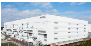
Yokkaichi Plant (Kioxia Corporation)
